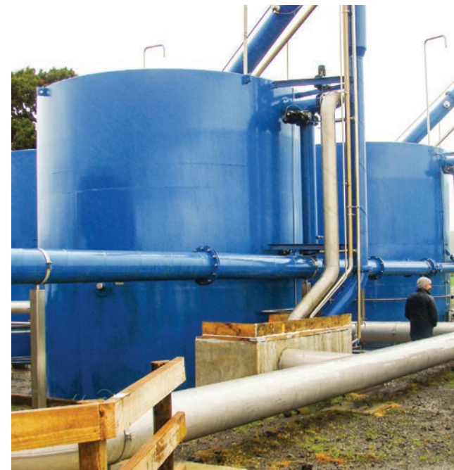
The Water filters painted bright blue.
