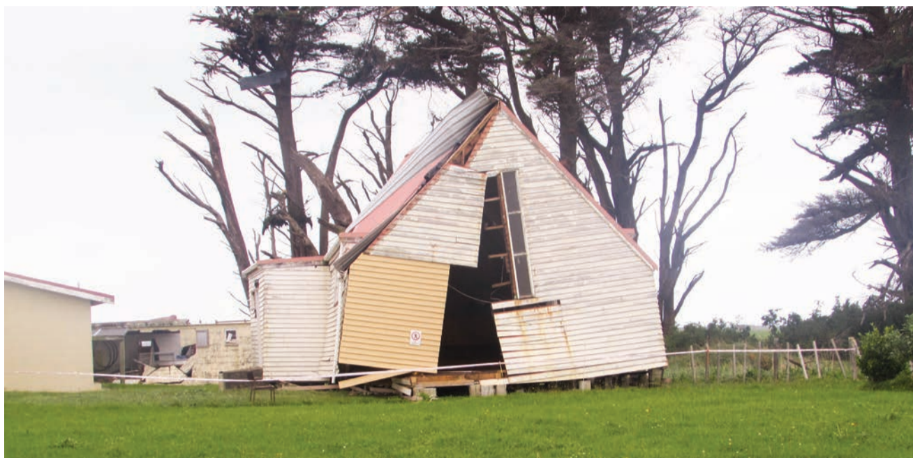
The chapel next to the Orimupiko Marae was extensively damaged in a storm last week.
